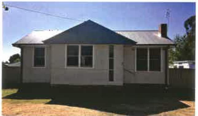
A Moama property has received a significant upgrade in 2018.
