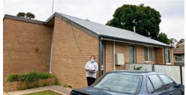
Deniliquin Client Officer Tash in Laman Crt, the property received a new Colourbond Roof as part of the Capital Works Project, installed by local plumbing Co Mick Farley Plumbing.
